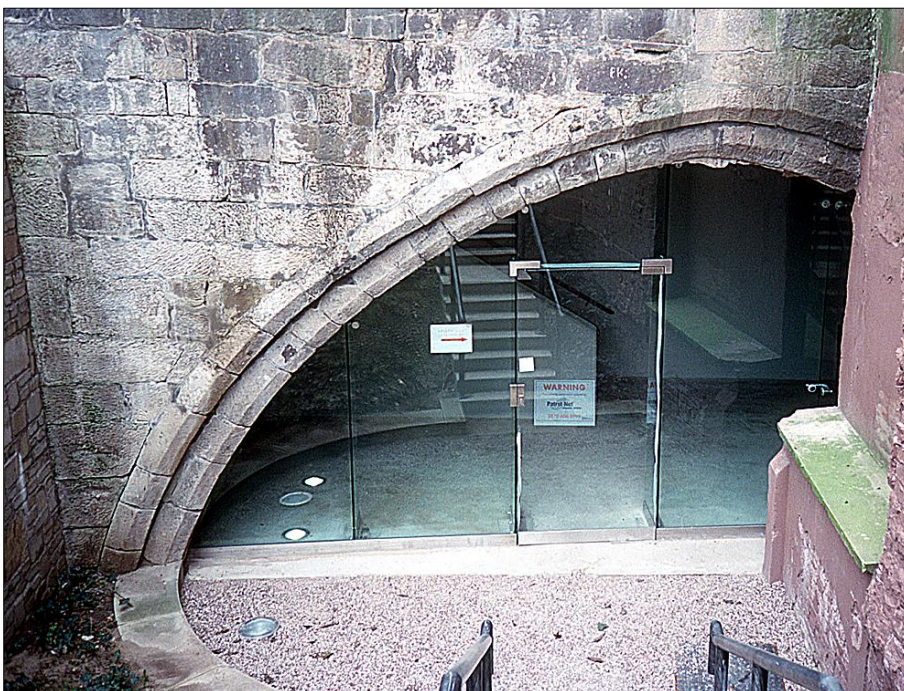
Ill B19: The western elevation of the north arch.
