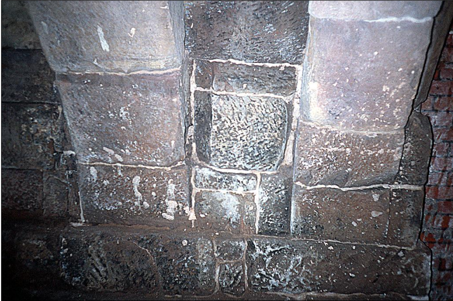
III B22: The south arch, detail of the south side, including a possible reused chamfered stone (centre).
