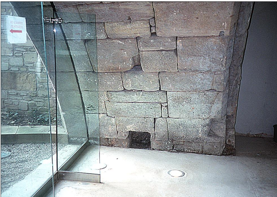
III B30: The north arch, the base of the north side.
