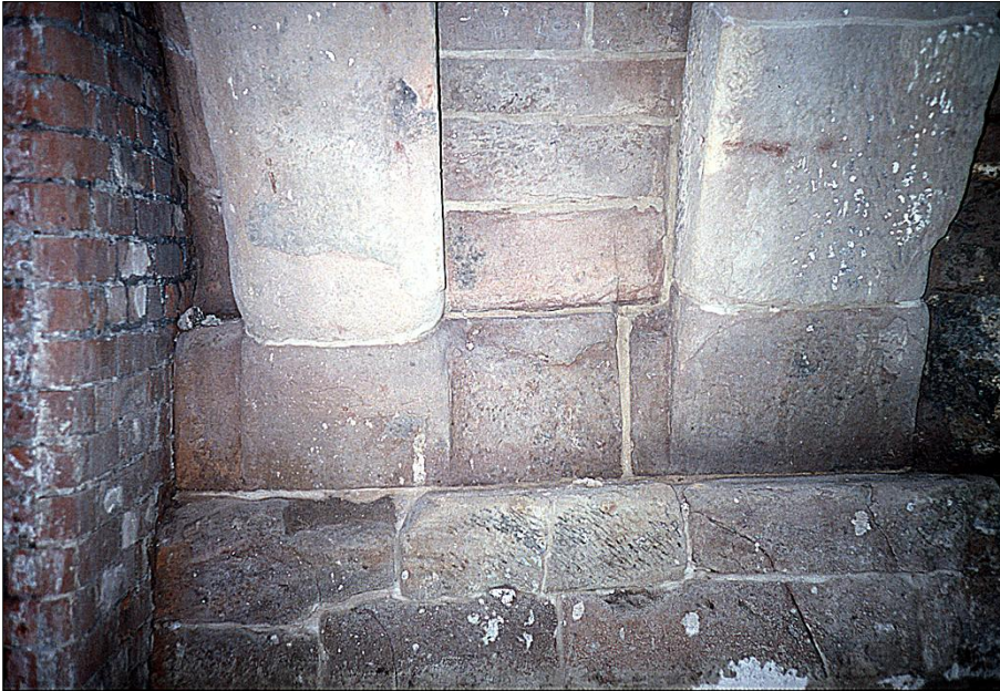
III B25: The south arch, north side, detail of the base of the central and western ribs.
