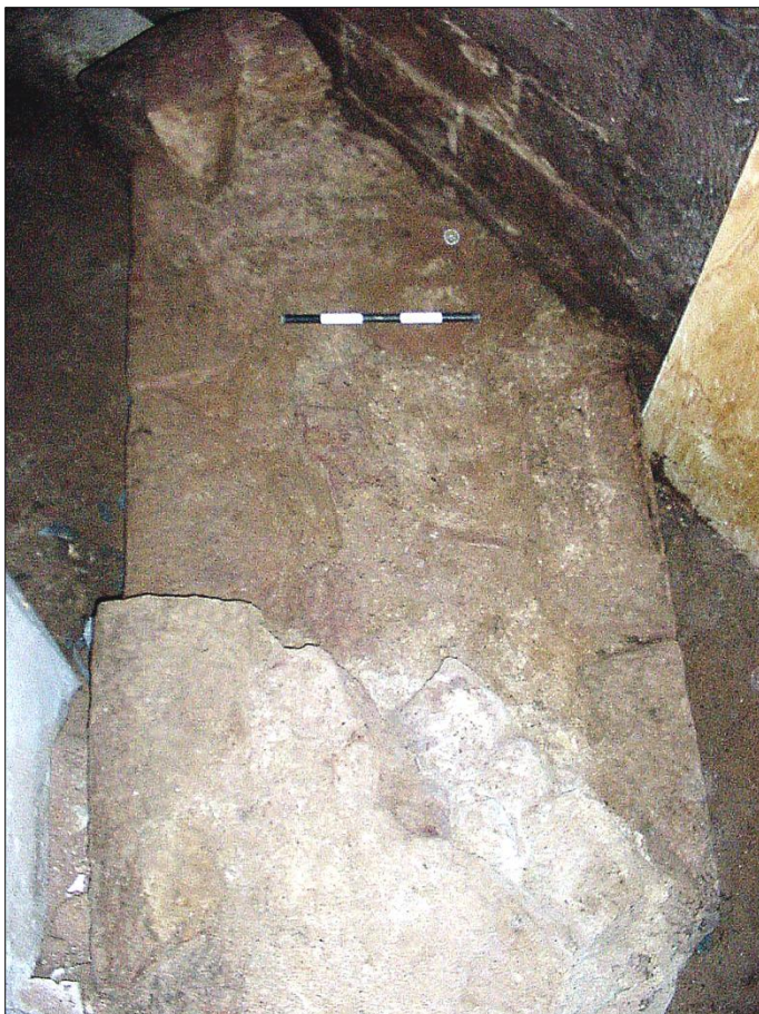
III B41: The 'cutwater', as reduced in height, viewed from the north-east.
