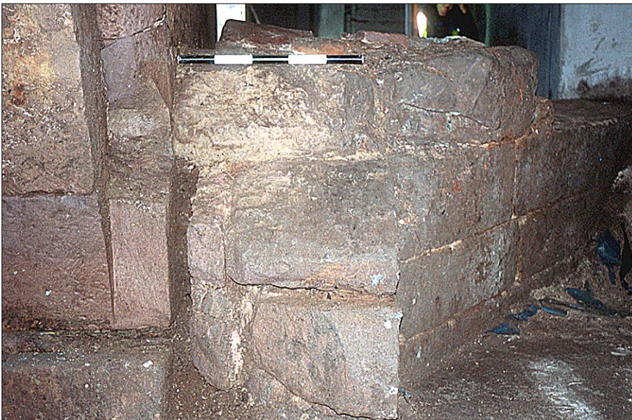
III B40: Detail of the 'cutwater', from the south, following the removal of the upper material. A silty fill is visible between the 'cutwater' and the bridge.
