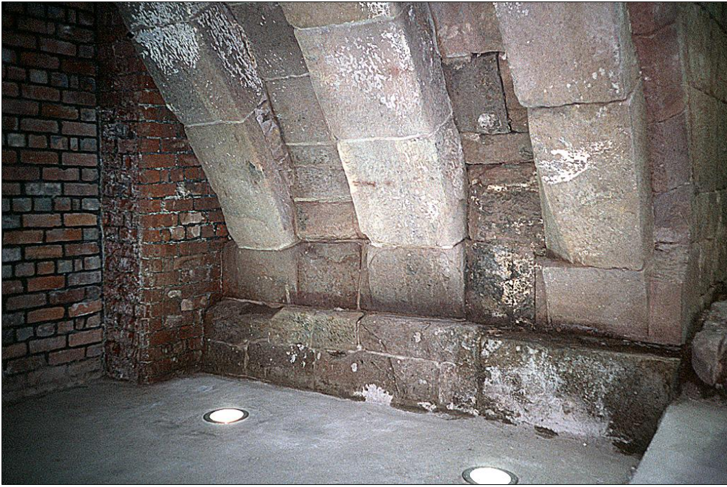
III B24: The south arch, the base of the north side.
