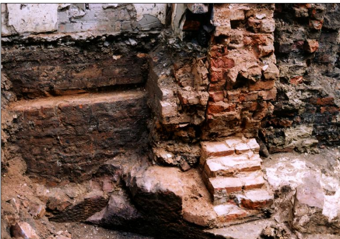
III B37: The western end of the 'cutwater', overlaid by the walls of Hanging Bridge Chambers (left) and Nos 10-12 Cateaton Street (left).
