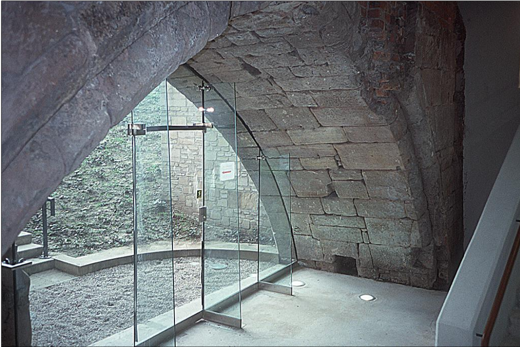
III B29: The north arch, viewed from the south-east.
