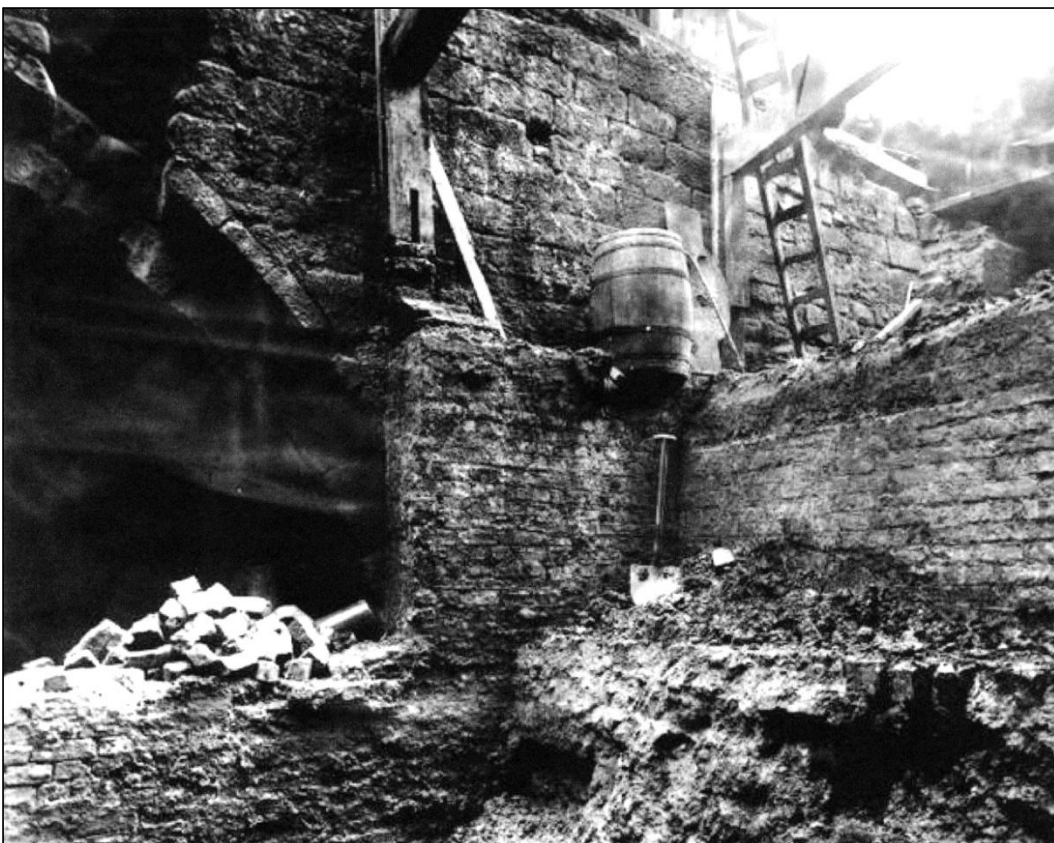
III B47: The south abutment of the bridge, 1890 (© Manchester Libraries).
