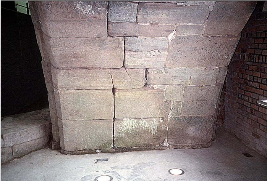
III B28: The north arch, the base of the south side.
