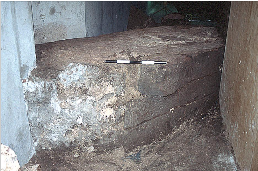
III B39: The 'cutwater', viewed from the north, following the removal of the upper material.
