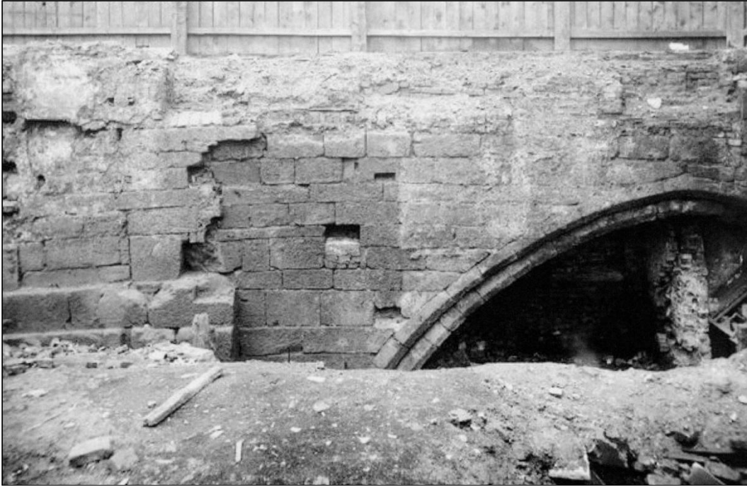
III B48: The north arch and abutment of the bridge, with the possible earlier buttress (left), 1900 (© Manchester Libraries).
