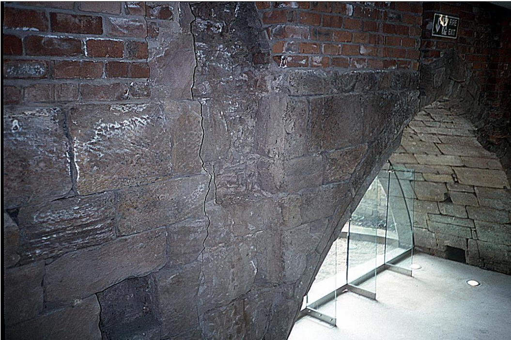
III B34: Detail of the east elevation, showing the vertical groove cut into the stonework above the central pier.
